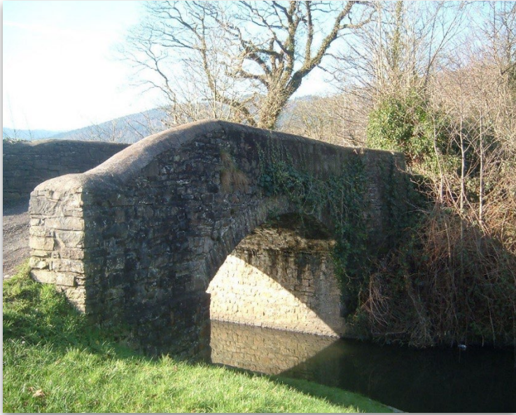
Bridge, Vale of Neath Canal near Rheola, Resolfen.
